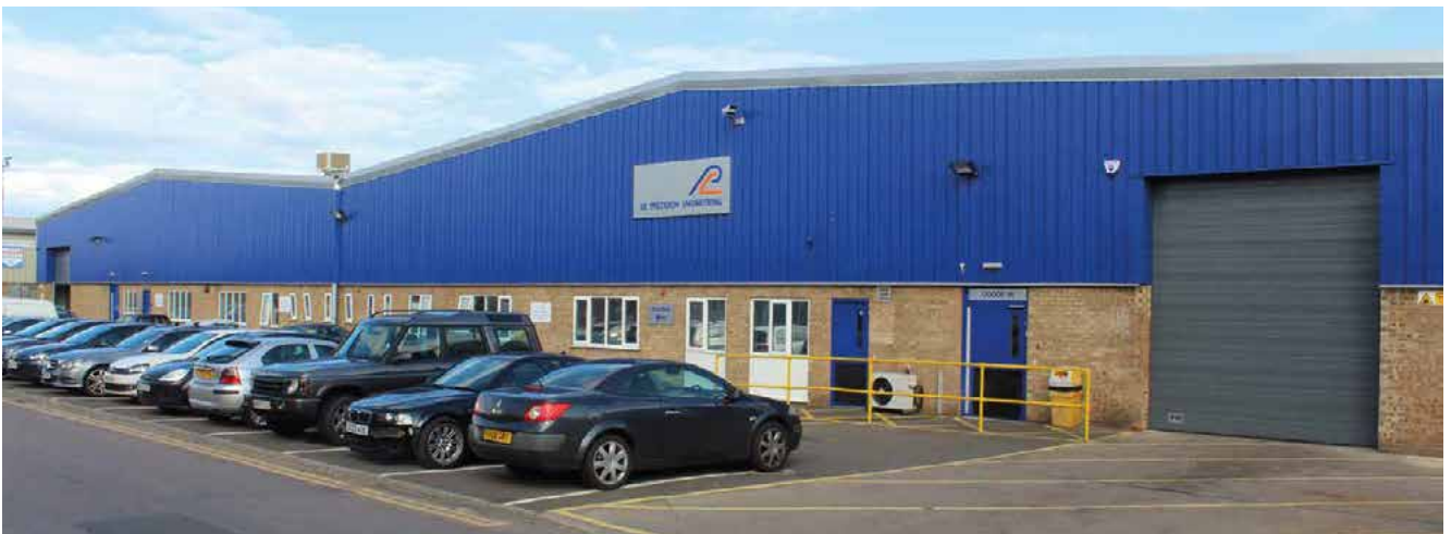
New headquarters on St James Mill Road within the Enterprise Zone
